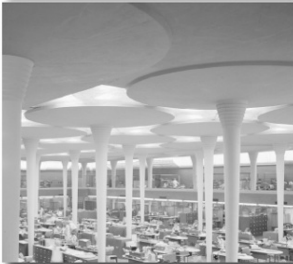
FIGURE 34 & 35. Johnson Wax Headquarters Building and Research Tower (above) and the Great Work Room of the Johnson Wax Building (left). Frank Lloyd Wright used concrete to create streamlined walls and wild "lily pad" columns. A dramatic field test conducted to demonstrate the weight-bearing capacity of the slender columns confirmed that they could bear many times their specified loads.
