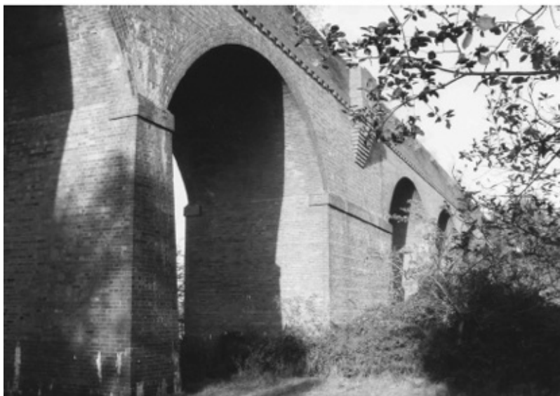
FIGURES 43 & 44. Views of the Hockley Viaduct in England. The structure was built of unreinforced concrete in the 1880s and, given minimum protection and maintenance, may last thousands of years.
