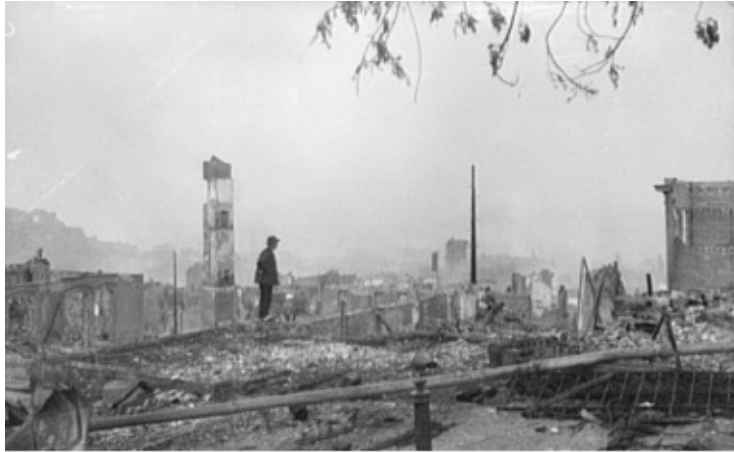
FIGURE 40. A man walking across the rubble caused by the 1906 disaster. Rubble photos were used by the concrete industry to show the “failure” of masonry buildings in the catastrophe. In fact, it was the reinforced concrete buildings in San Francisco that proved to be the most vulnerable in the earthquake and the subsequent fires.
