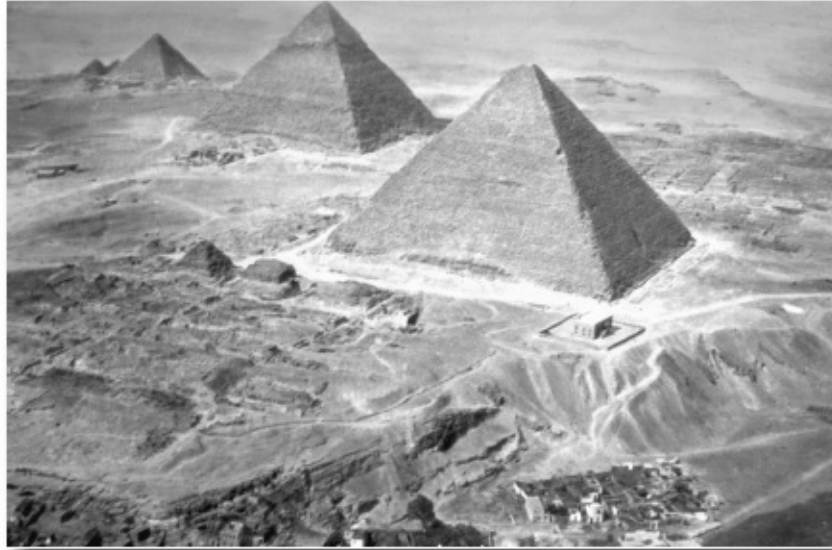
FIGURE 6. Aerial view of pyramids at Giza; the Great Pyramid of Khufu is in the right foreground. There is a contentious controversy about the materials used for the Giza pyramids. Some authorities claim that, instead of limestone, a special concrete was poured into molds that formed the blocks used to construct them. If true, it would be the largest use of concrete before the construction of the Panama Canal in the early twentieth century.
