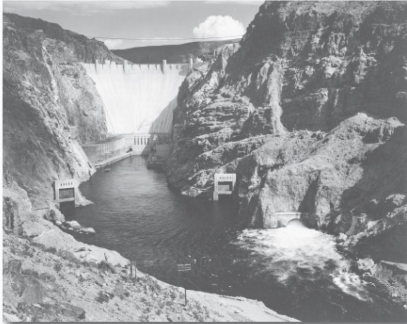
FIGURE 25. Hoover Dam In Arizona. So vast a quantity of concrete was used in its construction that some of the material is still curing—more than seventy-five years after the dam was dedicated in 1935!
