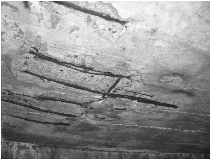
FIGURE 41. Disintegrating reinforced concrete floor slab. As the steel reinforcement bar oxidizes, its diameter dramatically expands, destroying the surrounding concrete as it, in turn, is destroyed by rust.
