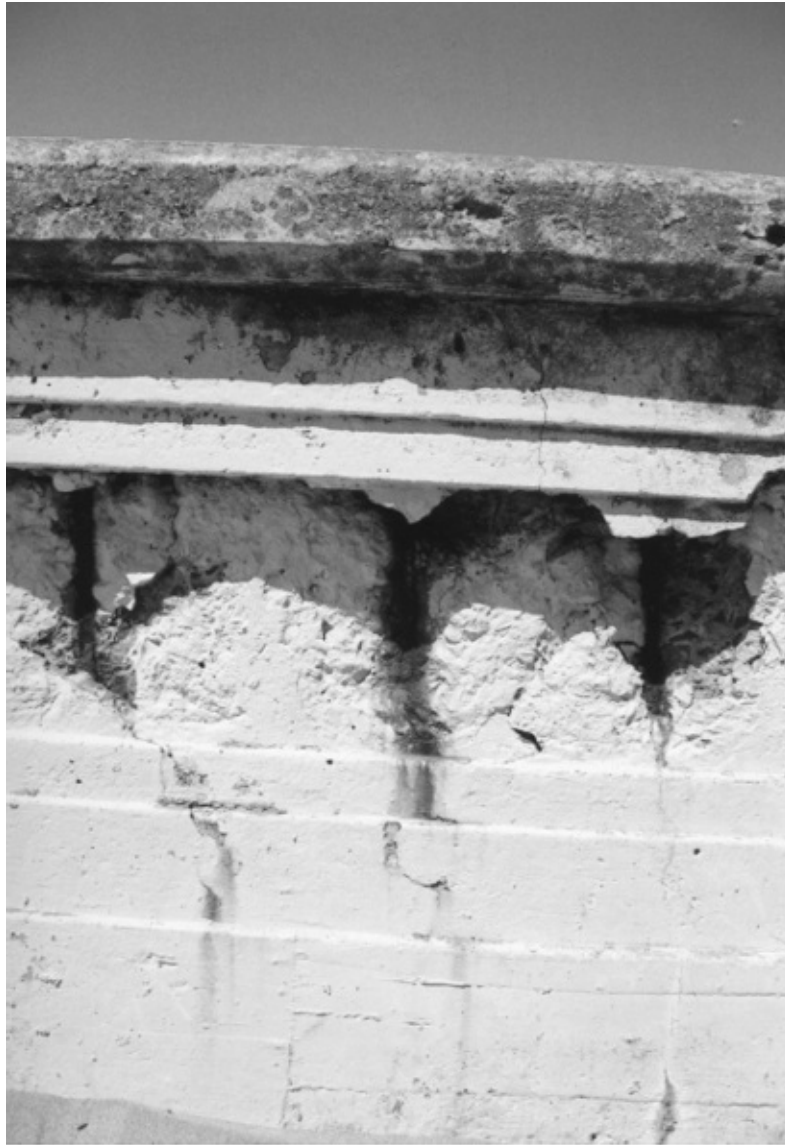
FIGURE 42. Disintegrating concrete wall. The middle stripe is merely a rust stain, the rebar itself having already vanished through oxidation. Once a certain corrosion point is reached, repair is difficult or impossible, and the structural integrity of the building is severely compromised.
